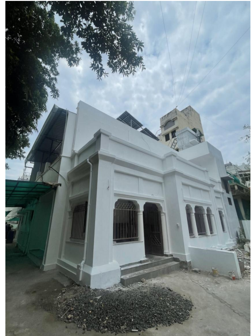
Site photograph: Waterproofing over 90 years old building at Nagpur, Maharashtra
