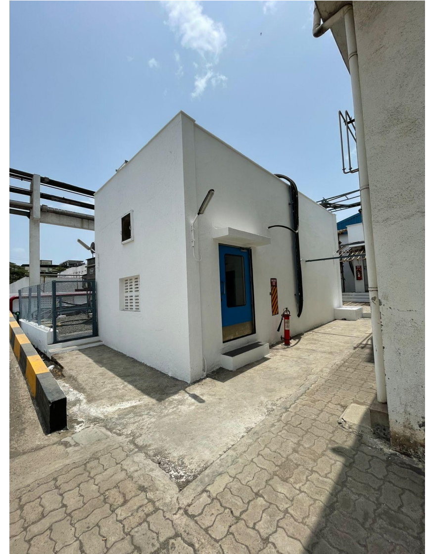
Site photograph: Control Panel Room, FDC Limited, Roha, Raigad, Maharashtra
